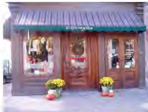
The awning on this structure helps to delineate the first story from upper floors. The building also presents a pleasant public face and provides visual interest.
