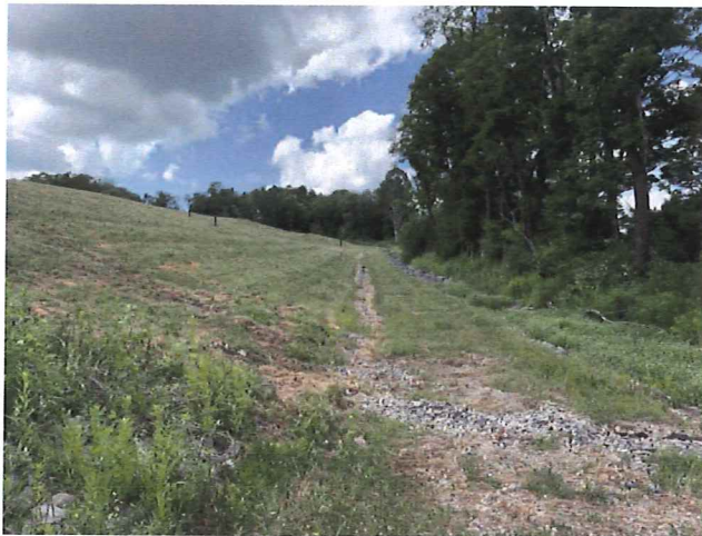
East side of the landfill.
