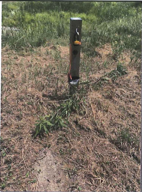
MW-2D appears to have been struck by the lawn mowing equipment.
