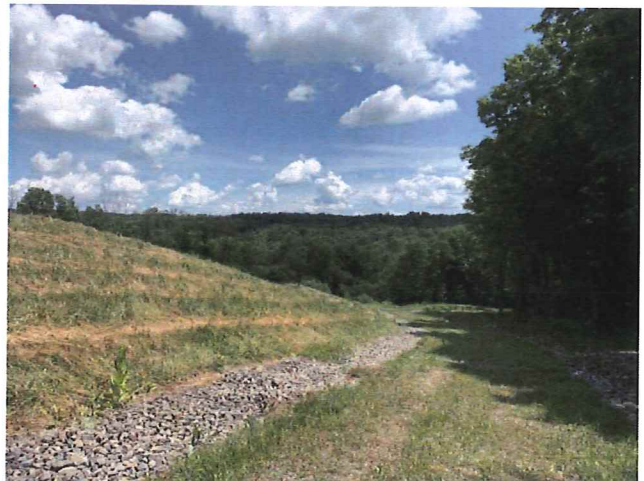
West side of the landfill.
