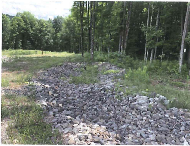
Drainage swale on the west side of the landfill.
