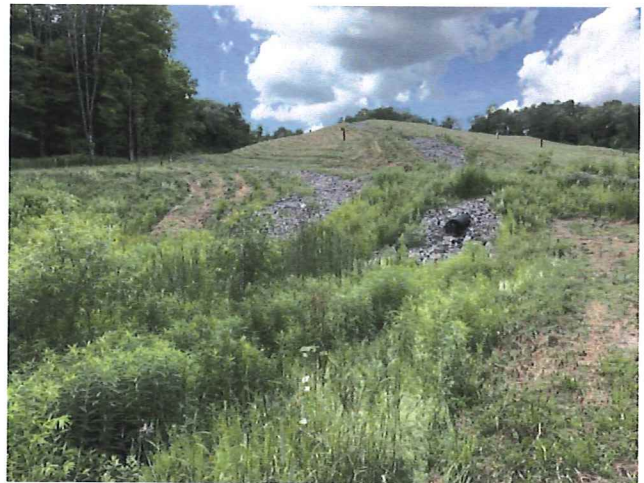
Drainage swale on the south side of the landfill.
