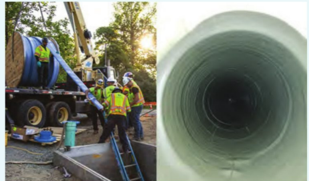
Thermal and UV Cure Lining
